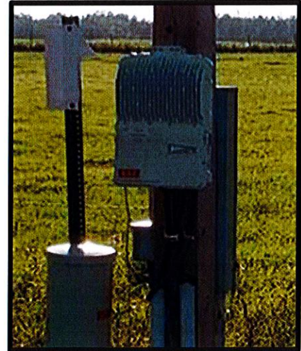
The DSLAM technology above gives old telephone phone lines a boost to make the data travel farther.
